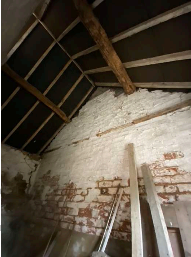
Fig 1 – inadequate ridge beam and rafters.
